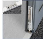
Concealed shoot bolts at the top and bottom of the inactive leaf hold the door securely in place. The adjustable keeps allow for easy alignment of the leaf position for a precise fit.
